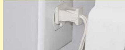
Pushing furniture against cords plugged into outlets
